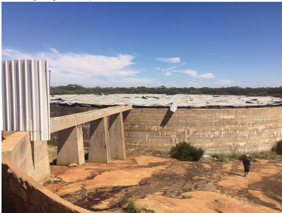
The current deteriorated state of Beringbooding Tank roof
